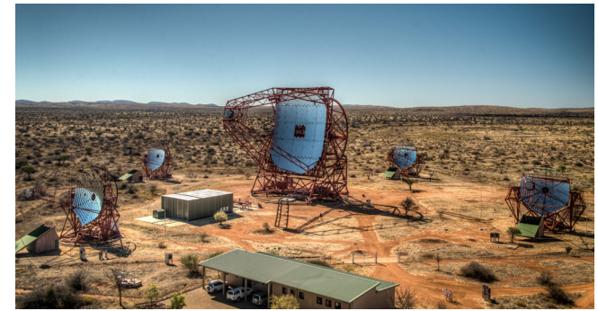
The High-Energy Stereoscopic System H.E.S.S.. The four smaller telescopes span a square of length 120 metres, in the centre of which the fifth, huge telescope is placed.
